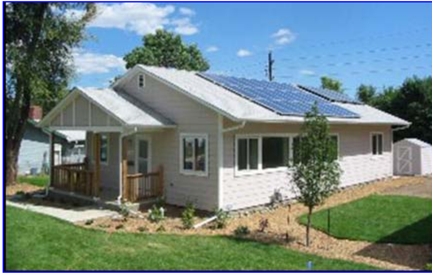
Figure 2. Completed NREL/Habitat Zero Energy Home (Credit: Pete Beverly)
