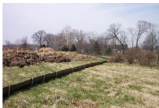
Silt fence installed at construction site Source: U.S. EPA. 2008. NPDES, Construction Site Stormwater Runoff Control
